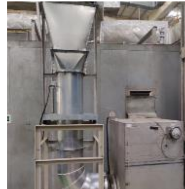
After- high efficiency Electronically Commutated motor installed in AHU
